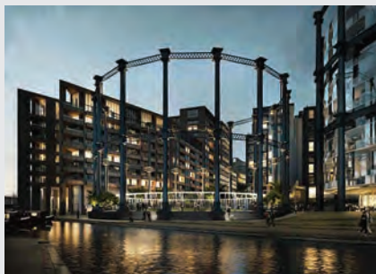
King Cross T1 Building, London, United Kingdom
