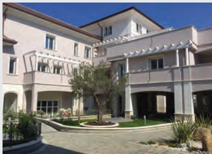
S. Rocco's Gardens Residential Estate, Seregno (MI), Italy
