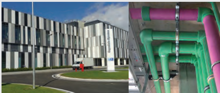
New Hospital Apuano, Massa Carrara, Italy
