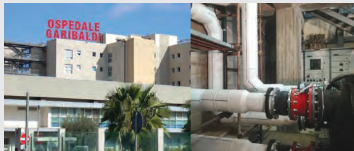
Garibaldi-Nesima General Hospital, Catania, Italy
