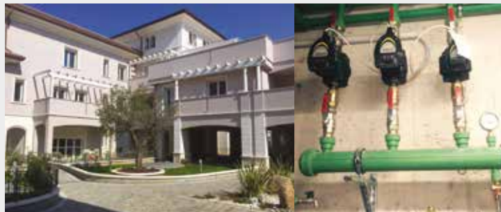
S. Rocco's Gardens Residential Estate, Seregno (MI), Italy
