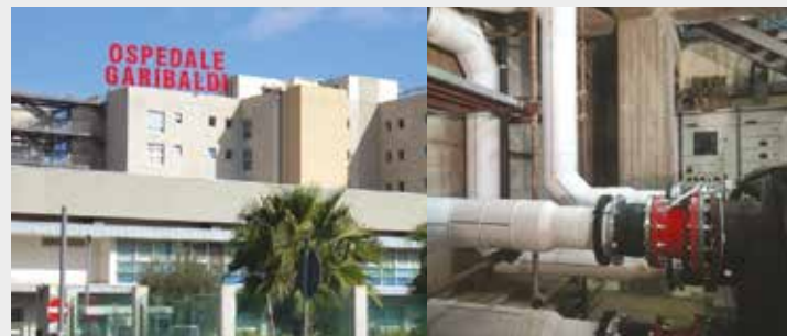
Garibaldi-Nesima General Hospital, Catania, Italy
