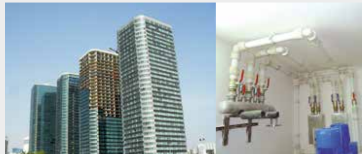
Bahia Center Residential Estate, Oran, Algeria
