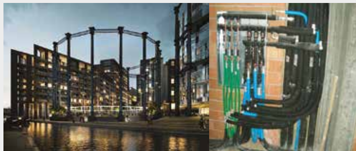
King Cross T1 Building, London, United Kingdom
