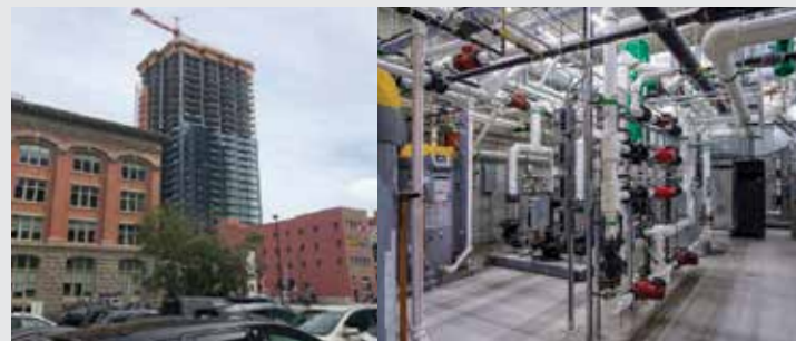
Upten Building, Calgary, Canada
