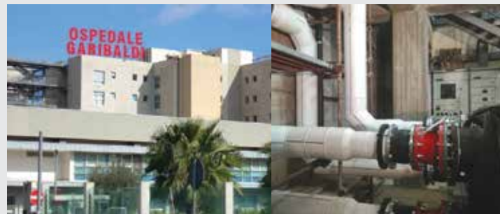
Garibaldi-Nesima General Hospital, Catania, Italy
