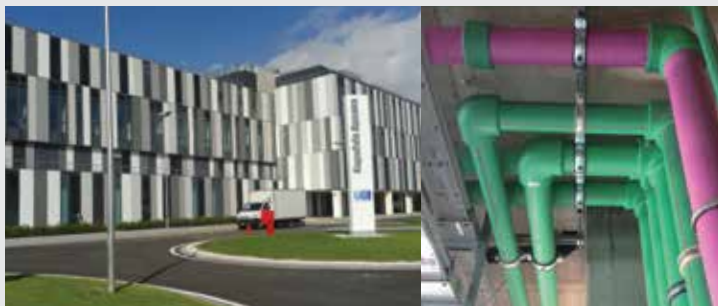
New Hospital Apuano, Massa Carrara, Italy
