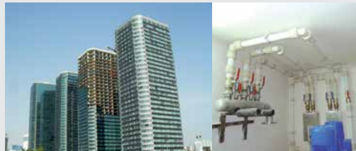
Bahia Center Residential Estate, Oran, Algeria
