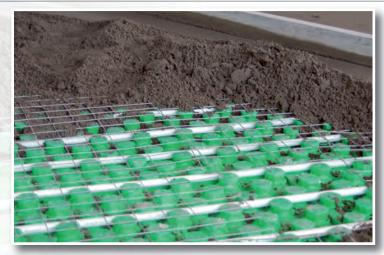
The insulating sheets are buried into the screed; the pipes will be installed on such sheets and will contain the water conditioning the surrounding thanks to the principle of heat exchange by radiation.
